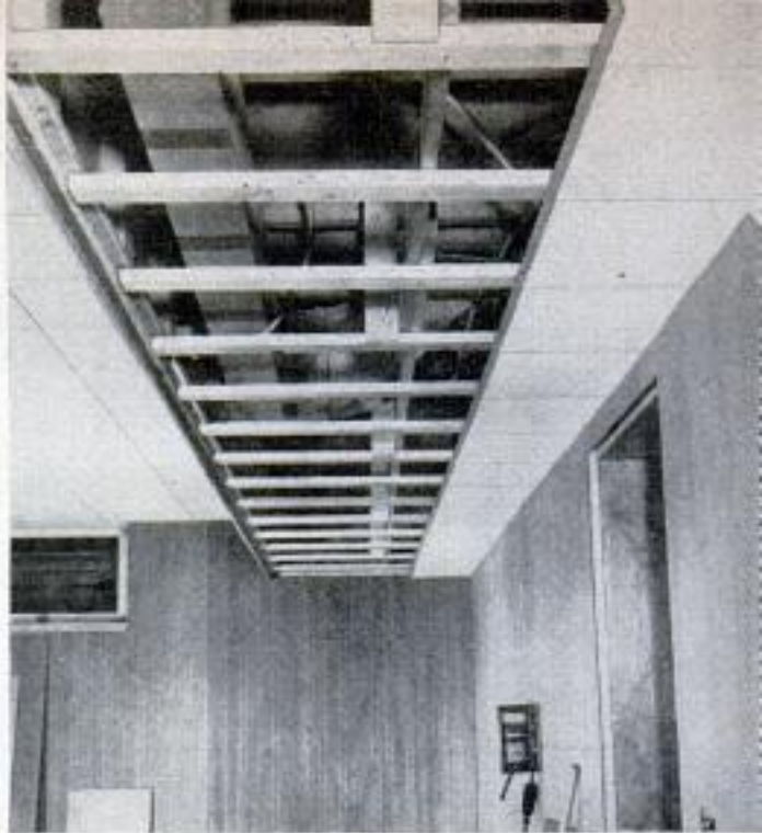
Boxing along both sides of room is used to conceal ducts and water pipes without lowering entire ceiling
